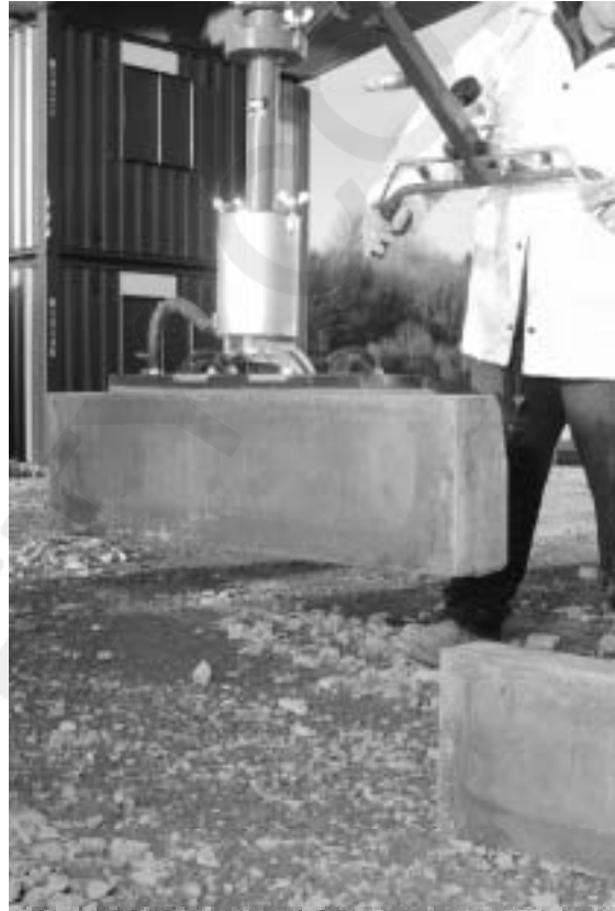
Figure 1 Handling kerbs using a vacuum lifter
