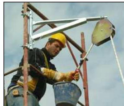
The load applied to the rope tends to make go up the slack side of the rope. When the slack side of the rope is vertical, it involves with him the brake, which then exerts an effort of wedging on the rope, which blocks in position.
