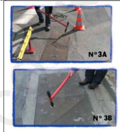
4) Commence by lifting out an end plate. To do this, position machine in front of or as near to the centre of gravity of the plate concerned, lift and roll.
