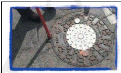
**5)** Position handle-bar shaft so as to have the greatest leverage.
