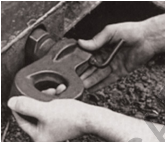
Figure 1 - Offer lug into slot. Left hand bottom side shown.
