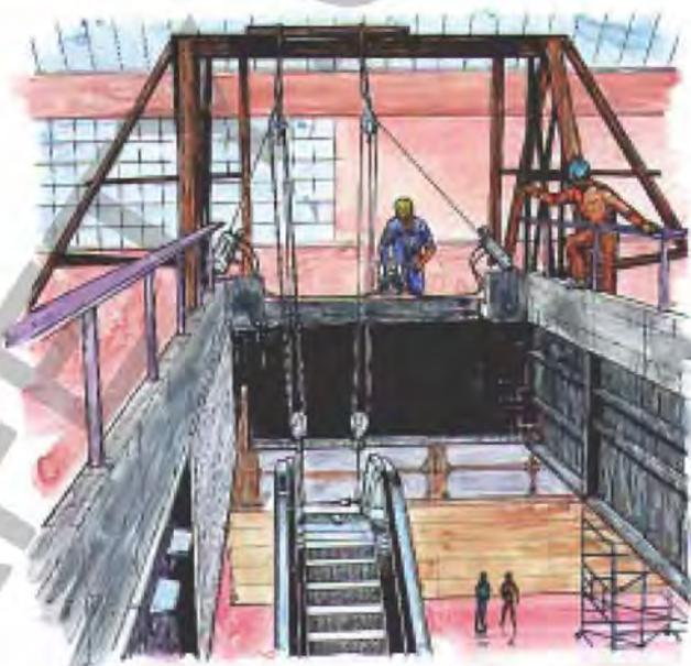
Fig. 27 - Installation of mechanical escalator (TU-16H)
