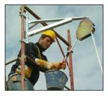
The load applied to the rope tends to make go up the slack side of the rope. When the slack side of the rope is vertical, it involves with him the brake, which then exerts an effort of wedging on the rope, which blocks in position.
