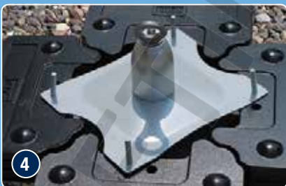
4 Set post and base onto the "L" bolts and plates
