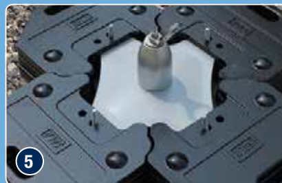
5 Install the remaining four plates and tighten bolts/nuts
